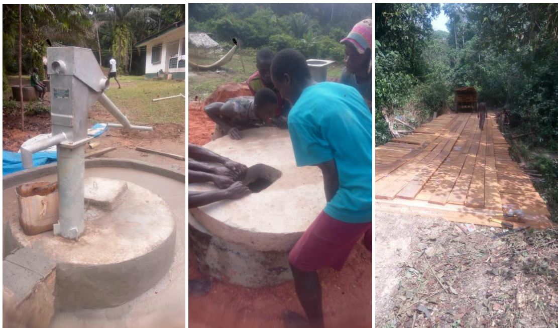
Hand pump construction at FDA headquarters (left) and Jalay Town (middle) for Sapo National Park and rehabilitated bridge at Grebo-Krahn National Park (right).
